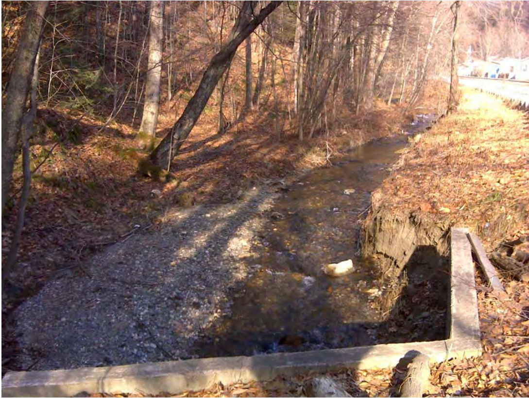
West of Black Mountain Road (near Crescent Drive) – facing north
