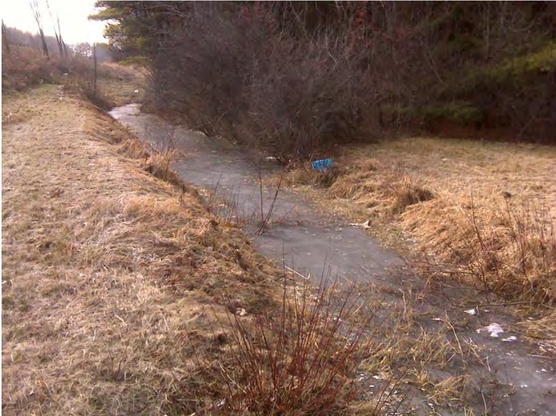
Southwest corner of I-91 and I-91 Chesterfield Road southbound ramps – facing south
