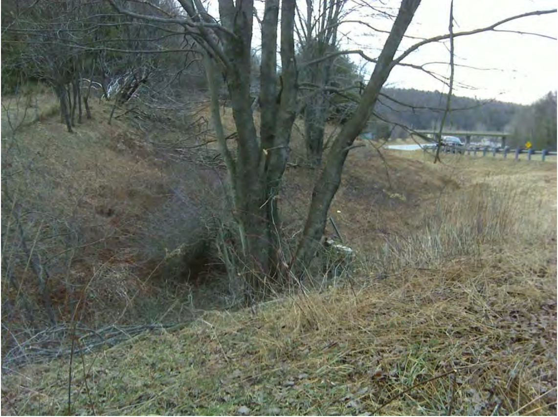
West side of I-91 (between Putney Road and I-91 Chesterfield Road ramps) – facing northeast
