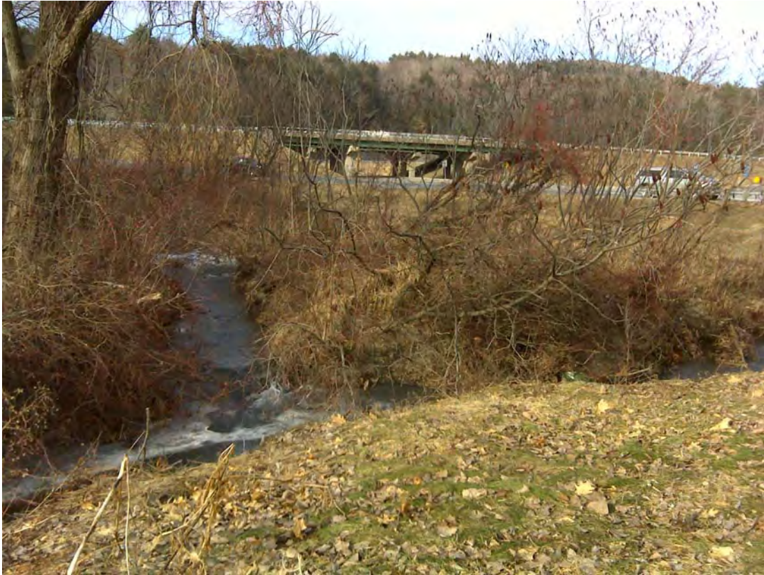
Southwest corner of Putney Road and Chesterfield Road – facing west
